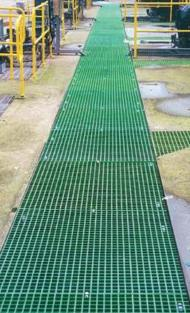
The proven gritted anti-slip surface of our moulded grating has one of the highest degrees of slip resistance ever measured for a walking surface, especially in wet, oily or frosty work areas. The integral gritted anti-slip top surface provides long-lasting slip resistant qualities. The material has excellent corrosion resistance, a factor which makes it a logical and cost-effective alternative to conventional steel materials.
